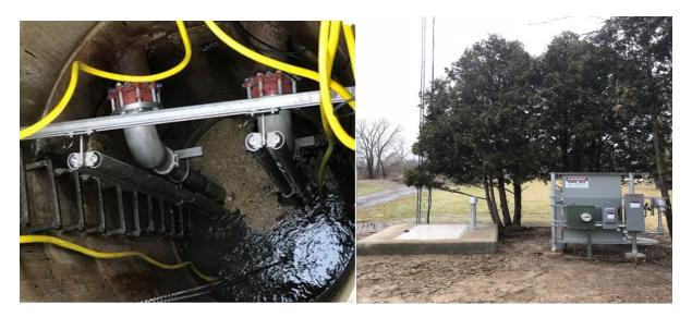
As you can see from the pictures, this rehab was a huge achievement, utilizing stainless steel hardware, aluminum hatches, and vented trays to allow fresh air to circulate to maximize corrosion resistances.
